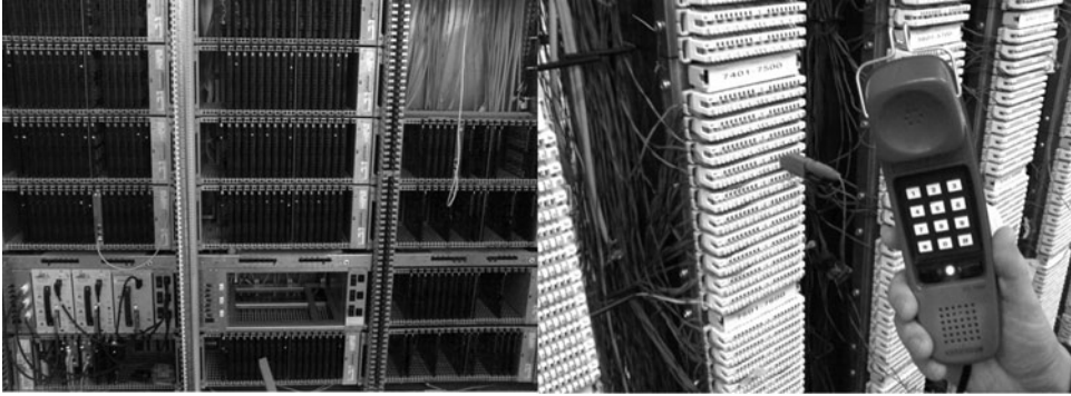
FIGURE 1.2 On the left, a switching board for about 3,000 subscribers; on the right, a red phone known as a “butt set” directly connected to listen in to an existing call.
